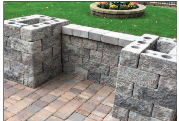
Install Wall Caps
