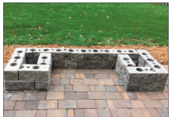
Completed 2nd Course
